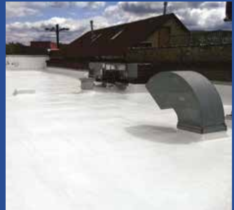
Liquid-Applied Roofing
